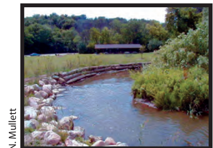
Middle Rouge River Stabilization
